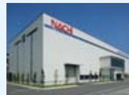
Special steel melting factory
