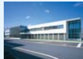
Internal broaches factory
