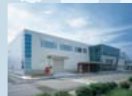
Hydraulic valves factory
