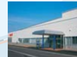
Bearing heat-treatment factory
