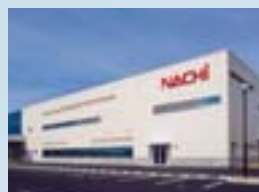
Parts processing factory
