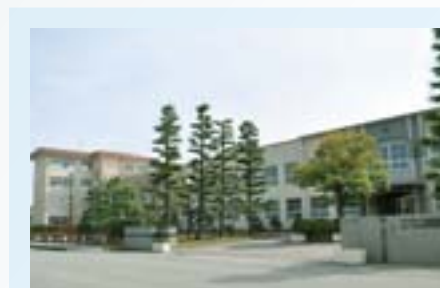
FUJIKOSHI Technical High School
